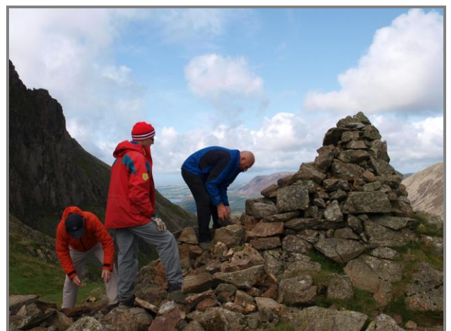
Rebuilding of Robinsons Cairn
