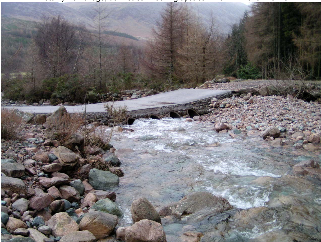
Photo 2) Irish Bridge, Photo from NY13233 13762, downstream.
