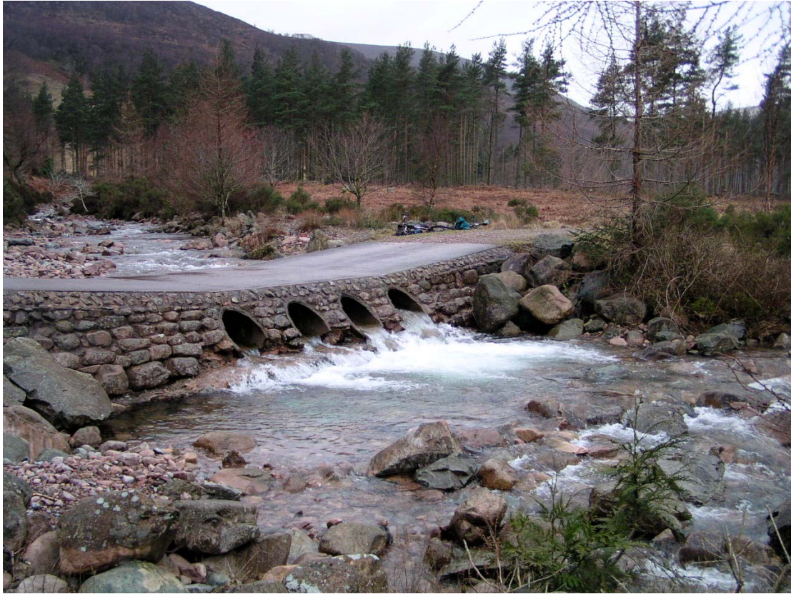
Photo 1) Irish bridge, downstream looking upstream from NY13257 13778
